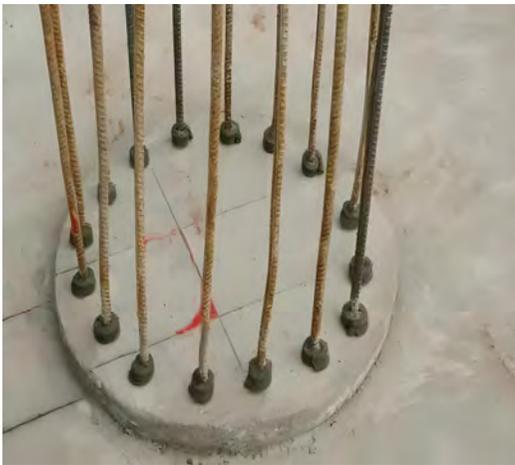
桩顶安装遇水膨胀止水条
